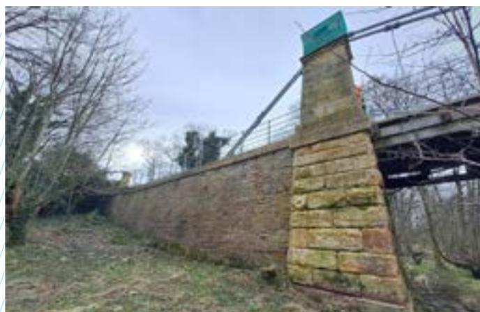
The masonry towers are in process of being covered with debris netting, mitigating any potential delay by protecting against nesting birds. Once the utility diversions are completed, scaffolding will be installed, and part removal of the towers will begin.
