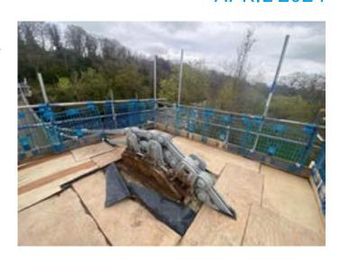
During the course of the project, the whole suspension and deck structure will be removed, refurbished and re-erected.
